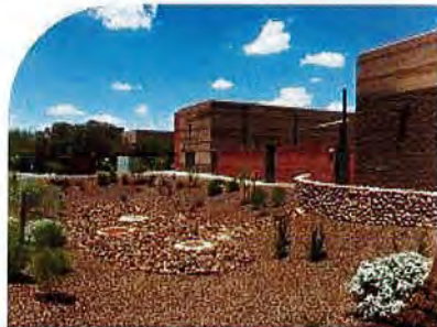
Underground storage of stormwater runoff may be allowed if approved by the SRPMIC Floodplain Administrator
