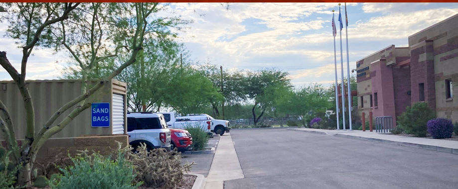
Station 294 (Indian School & Center St.) 11561 E. Indian School Rd. Scottsdale, AZ 85256
